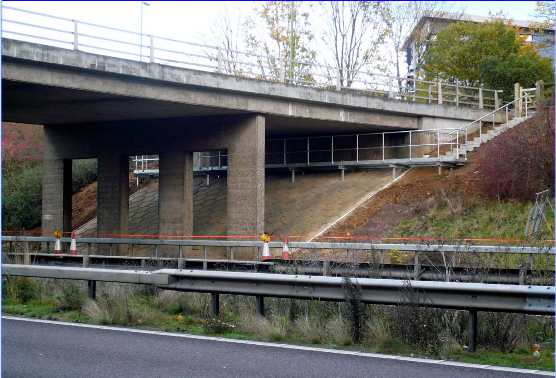
A1(M) Junction 7. 4 Modular Platforms & Stairways Installed by 6 Men in 10 Working Days
