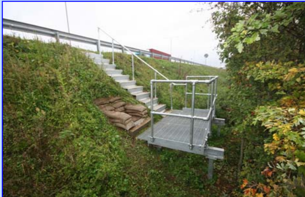
Installation of adjustable supports
