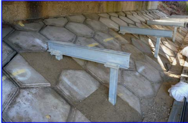
Installation of adjustable supports
